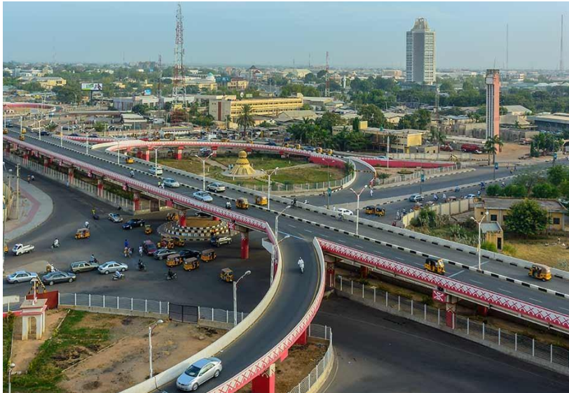
Murtala Mohammed Flyover Kano
